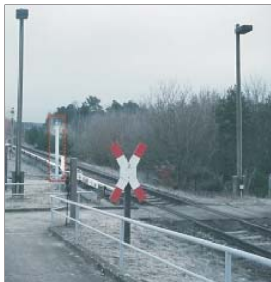
Fig. 3 • S-Bahn Berlin GmbH line S1 IR transmitter immediately next to the track
