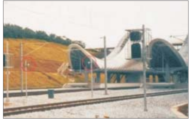
Fig. 6 • Express Rail Link KLIA in Kuala Lumpur IR transmitter immediately next to the track
